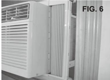
**3** Extend the side panels out against the window frame (FIG. 7).
